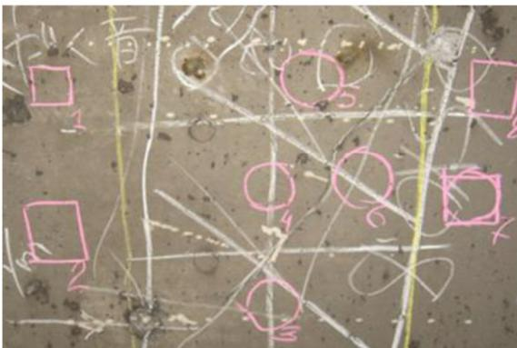
Fig. 27 Defect area in Shin-kansen tunnel.
